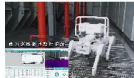
Converter Station Inspection in Zhejiang
